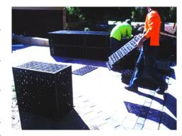
The Elite<sup>TM</sup> Polypropylene soakwell consists of a homogeneous polypropylene material exhibiting the same corrosion resistance throughout which eliminates the need for additional maintenance.
